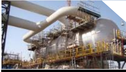
MEP for Bu Hasa Oil Project (Tecnicas Reunidas) AED 315 million
