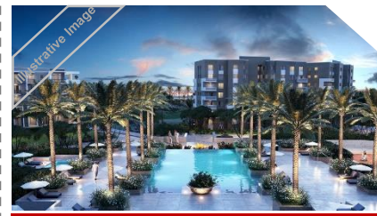
Construction of The Fourteen Golf Residences, Uptown Cairo, Egypt (Emaar Misr) AED 110 million
