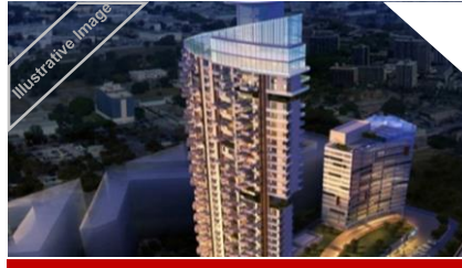
Construction of Navin Minar, India (Raheja Developers) AED 219 million
