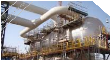
MEP for Bu Hasa Oil Project (Tecnicas Reunidas) AED 315 million
