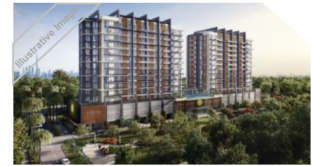
MEP for Wilton Park Residence (Ellington Properties) AED 192 million
